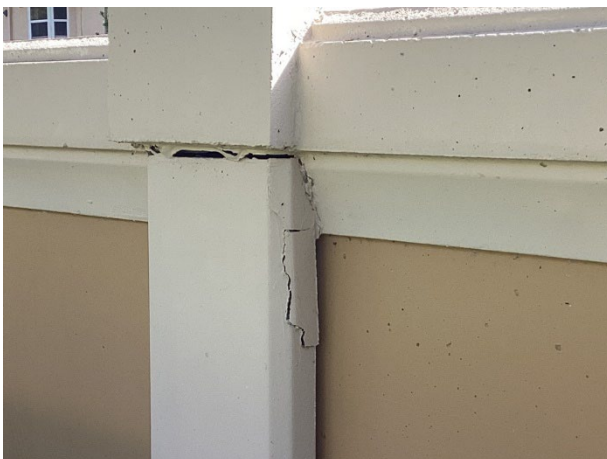
Wall stucco cracks
