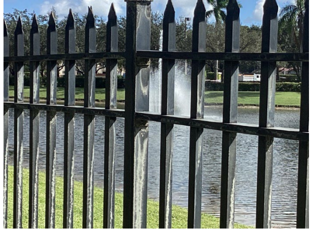
Fence finish deterioration
