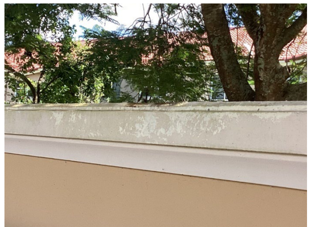
Wall paint finish deterioration
