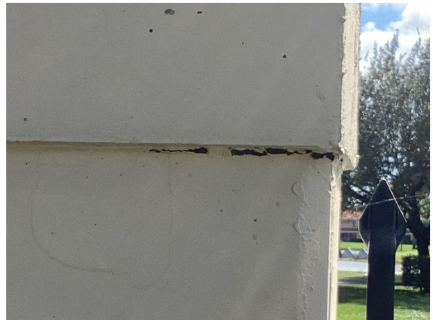
Wall stucco cracks
