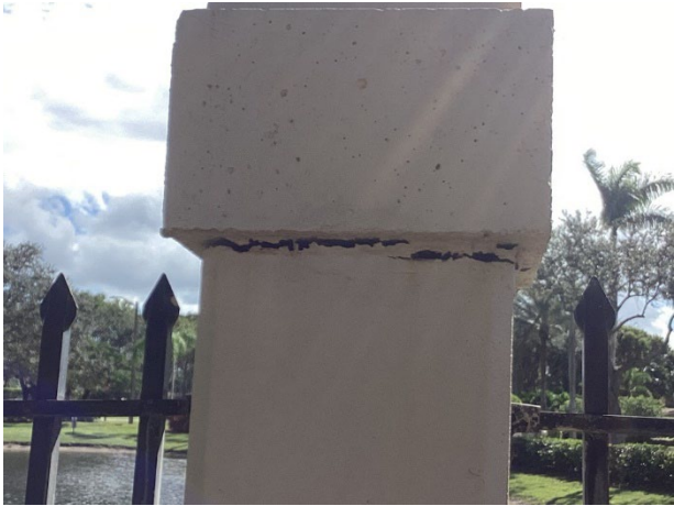
Wall stucco cracks
