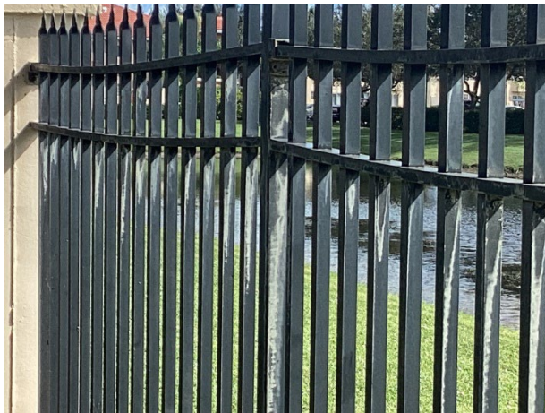
Fence finish deterioration
