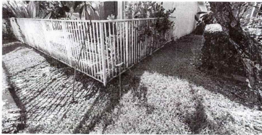
Orange Stake location of irrigation valve/leak
